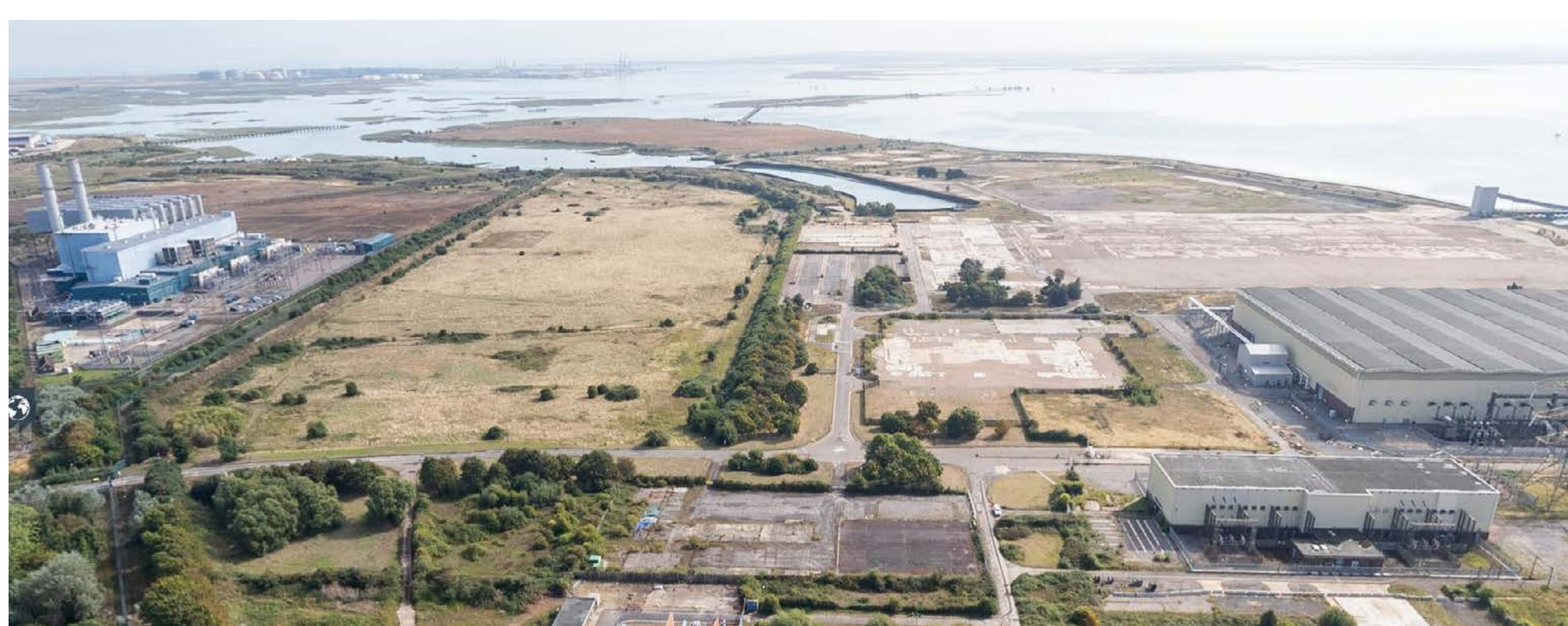
Photograph taken from the centre of the site looking East
